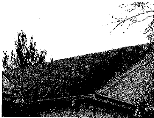
Asphalt shingles on pitched roof
